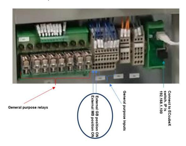
Note that an input is activated with potential free signal by shortening the two respective input terminals.
